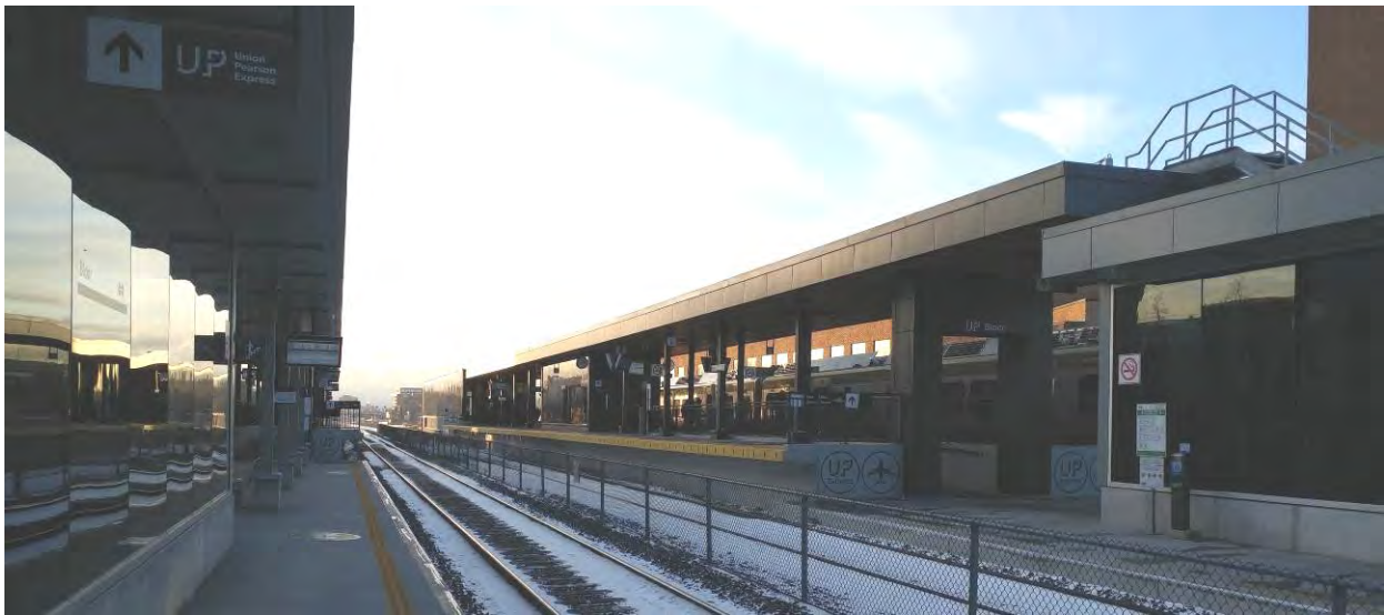
Figure 13-9: Example High Platform with Low Platform in the Foreground
